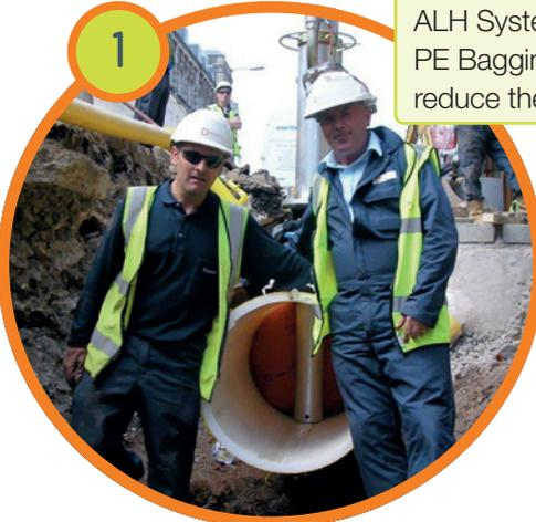
ALH Systems' Large Diameter PE Bagging-off equipment – to reduce the size of the drilling
