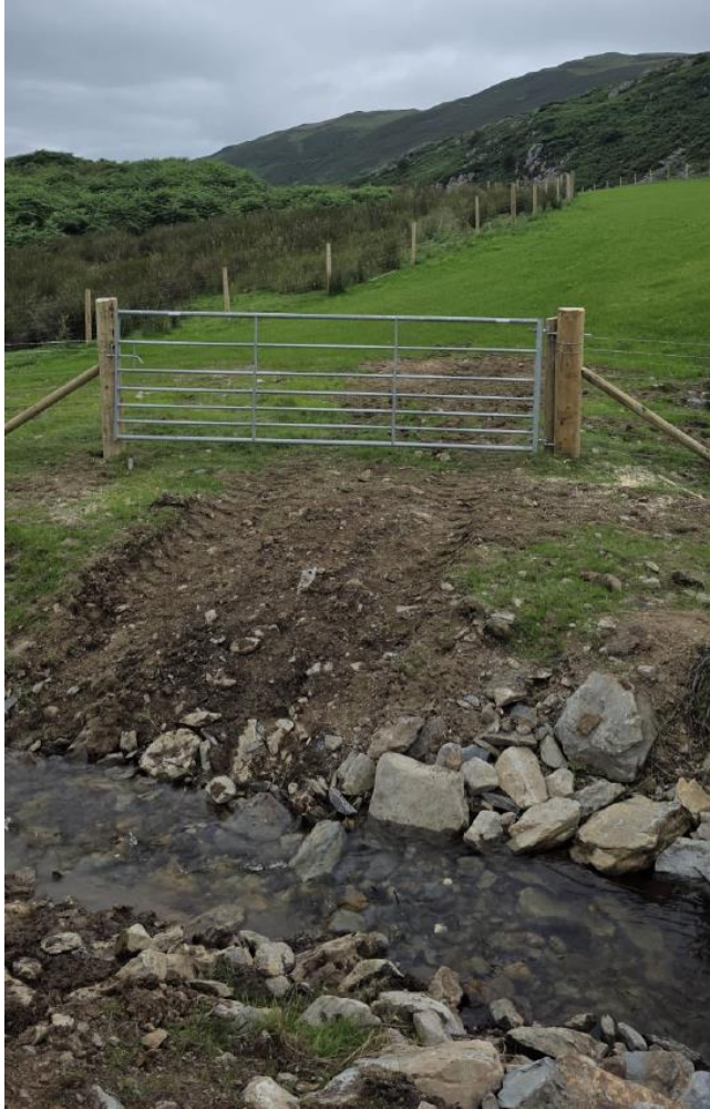
Permanent gate installation
