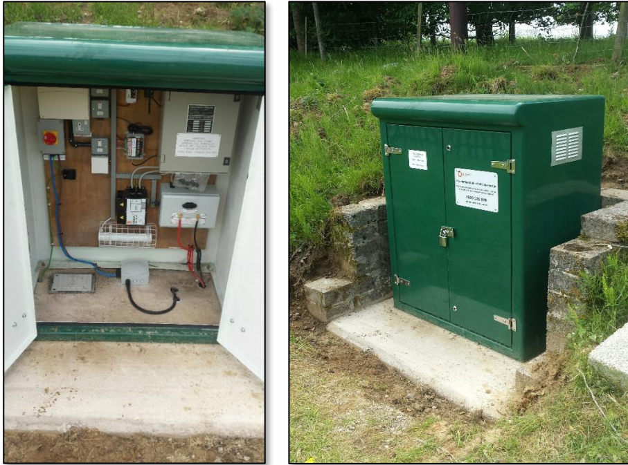
Figure 9 - Hinton Charterhouse TR after wholesale replacement
