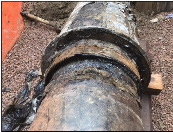
Figure 13 – Sleeve end seal replacement, before (1)
