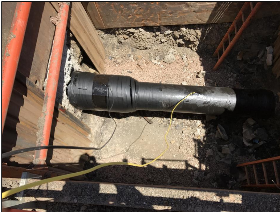
Figure 15 – Sleeve end seal replacement, after
