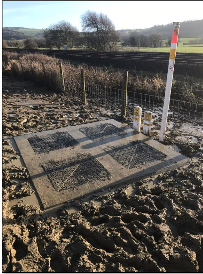
Figure 12 - Valve chamber replacement and valve/pipework refurbishment complete
