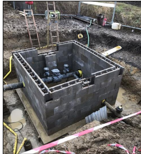
Figure 11 - During valve chamber replacement works
