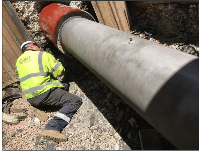
Figure 14 – Sleeve end seal replacement, before (2)
