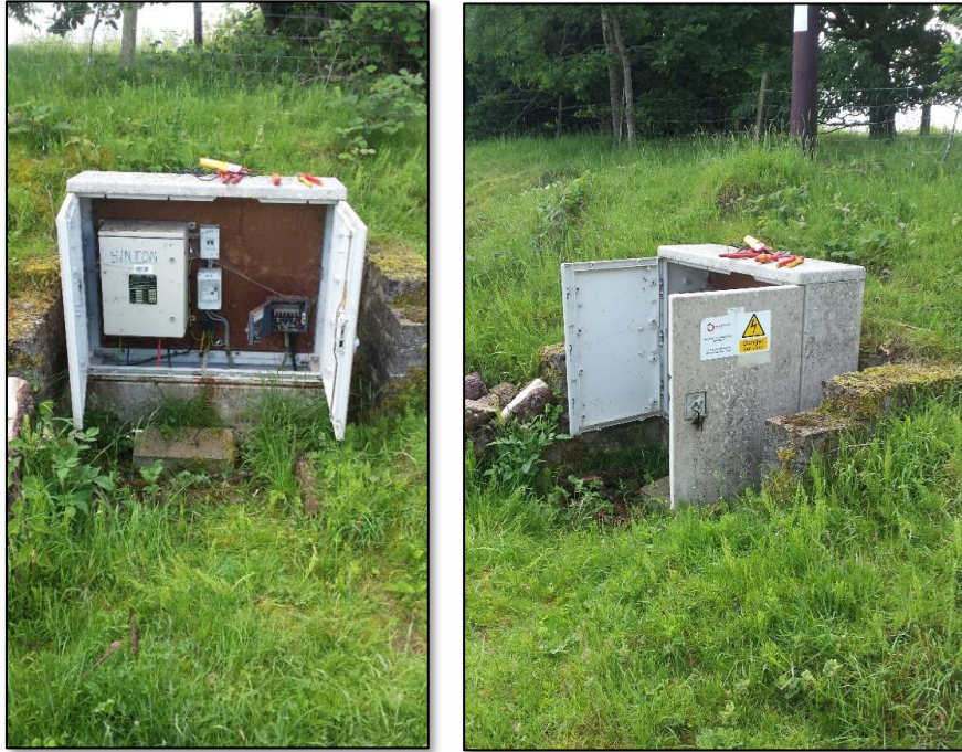
Figure 8 – Hinton Charterhouse TR before wholesale replacement
