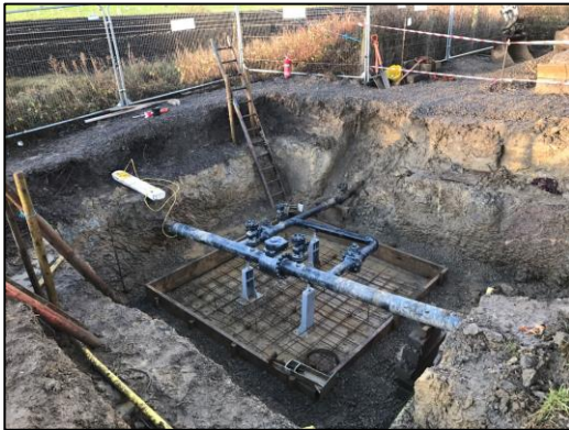
Figure 11 - During valve chamber replacement works
