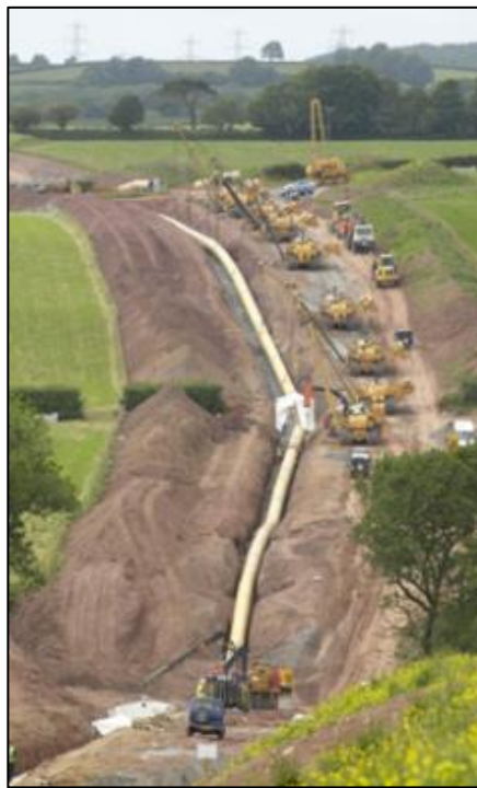
Figure 1 - LTS pipeline under construction
